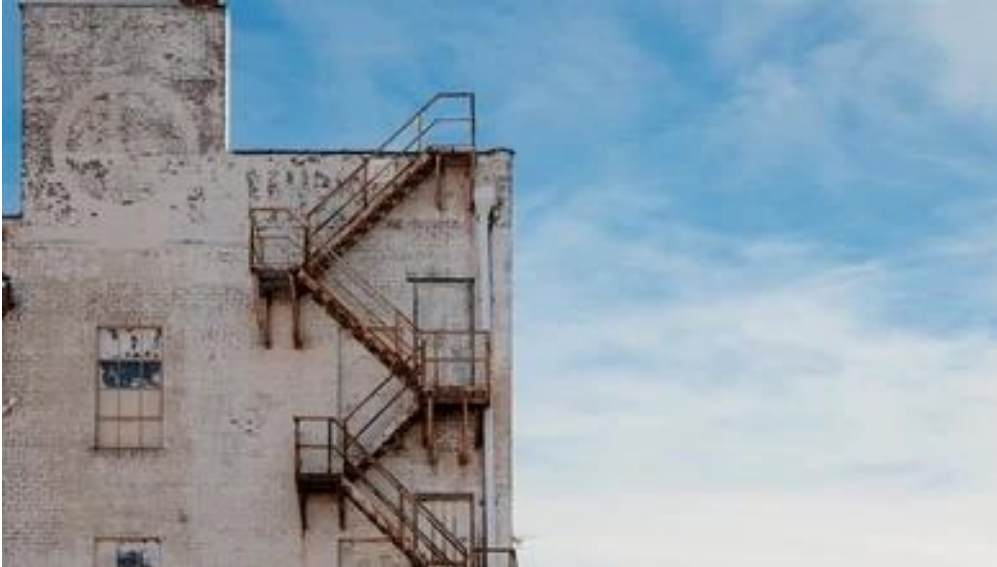
Fire external stair
