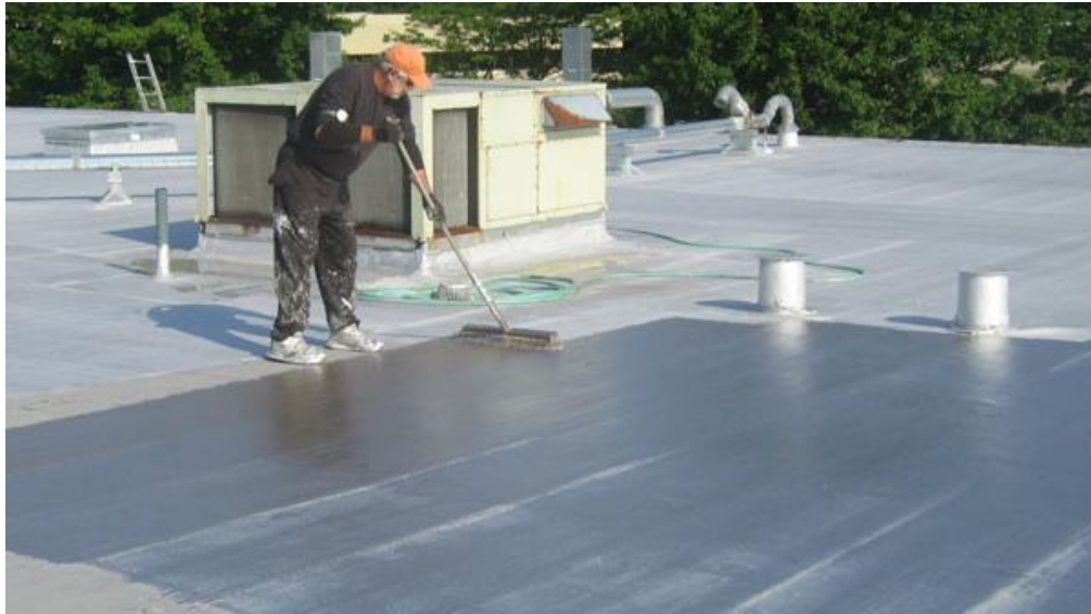
Reflective roof coating
