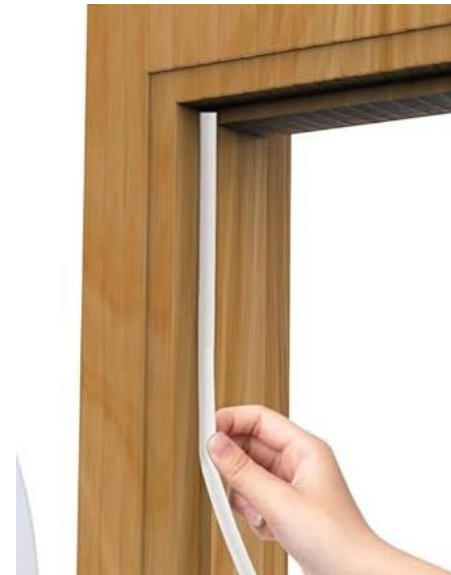
Air stripping and caulking
