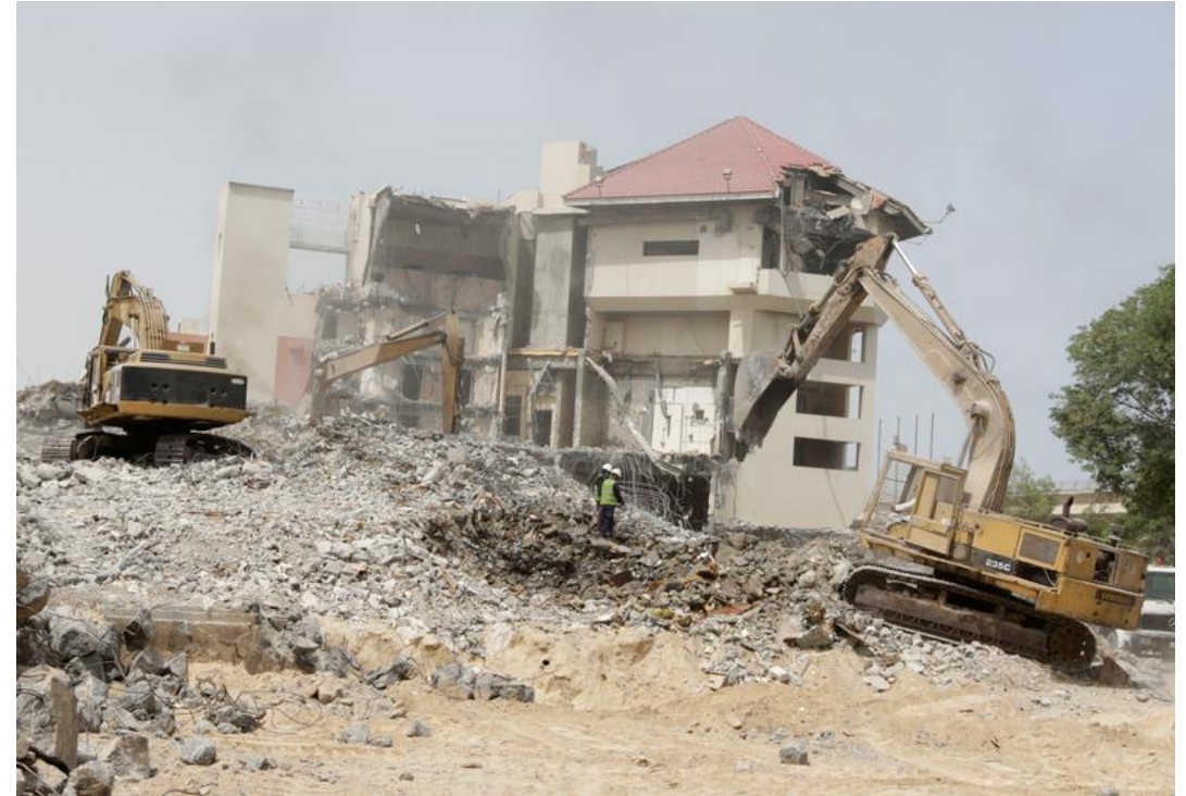
Demolition of Metropolitan hotel. Source: construction week online
