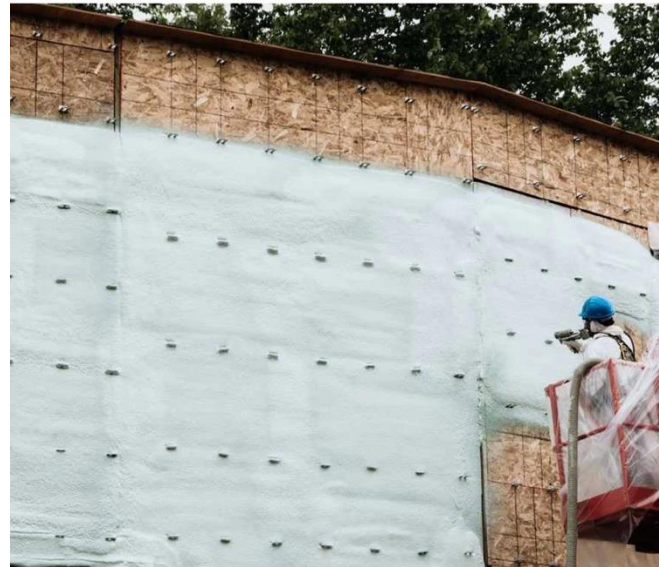
Spray foam insulation
