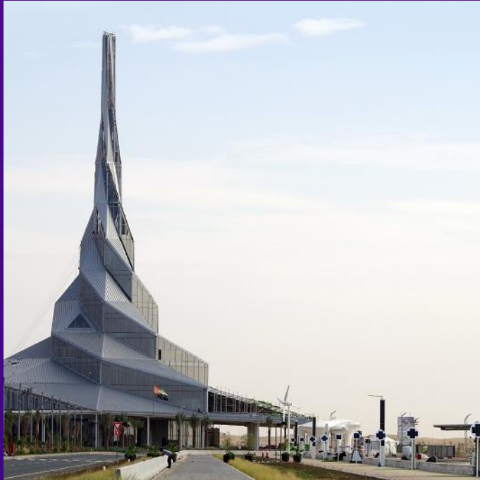
Mohammed bin Rashid Al Maktoum Solar Park
