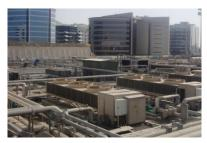
Client: Majid Al Futtaim Properties Location: Dubai, UAE Services provided: An Energy audit of the HVAC equipment was followed up by a detailed technical and economic feasibility study recommendations included replacing existing chillers and identified a range of solutions with paybacks between 7 and 11 years. Status: Complete 2014
