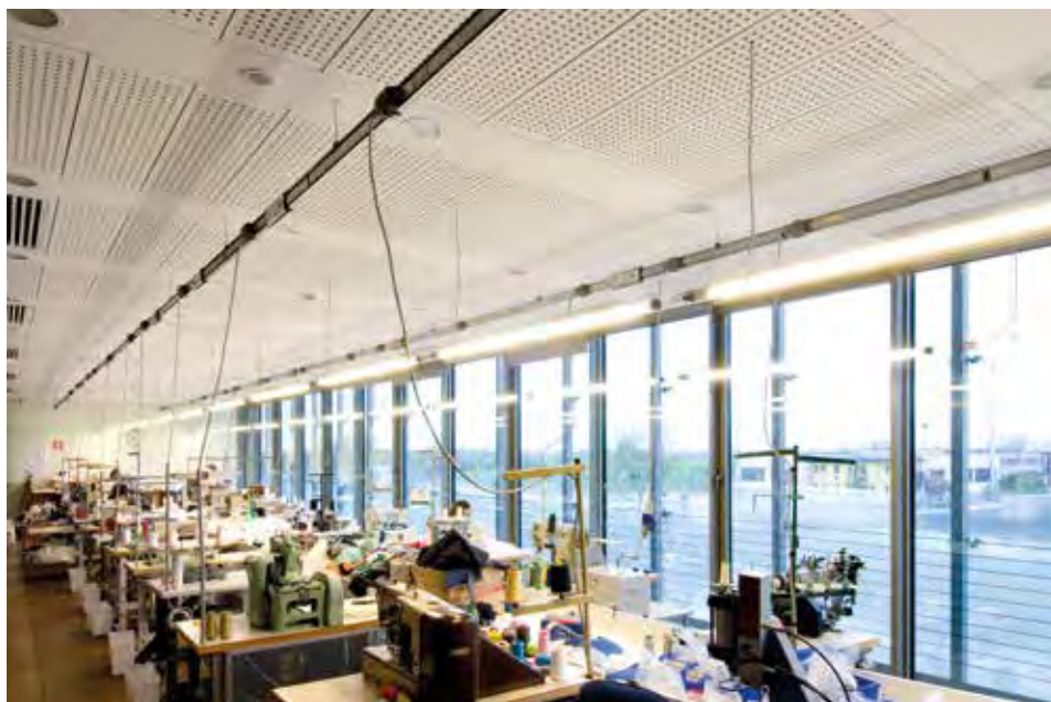
Example of lighting and small power distribution
